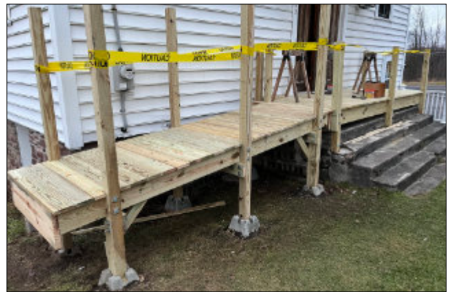
Figure 5: Entry platform and first ramp section under construction
