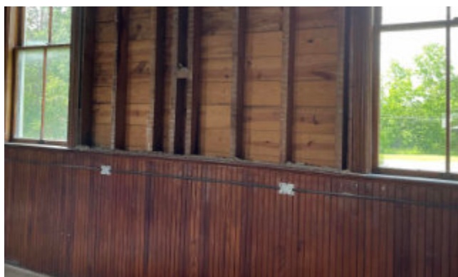
Figure 4: locating future electrical outlets
