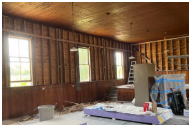
Figure 3: Lath board removal
